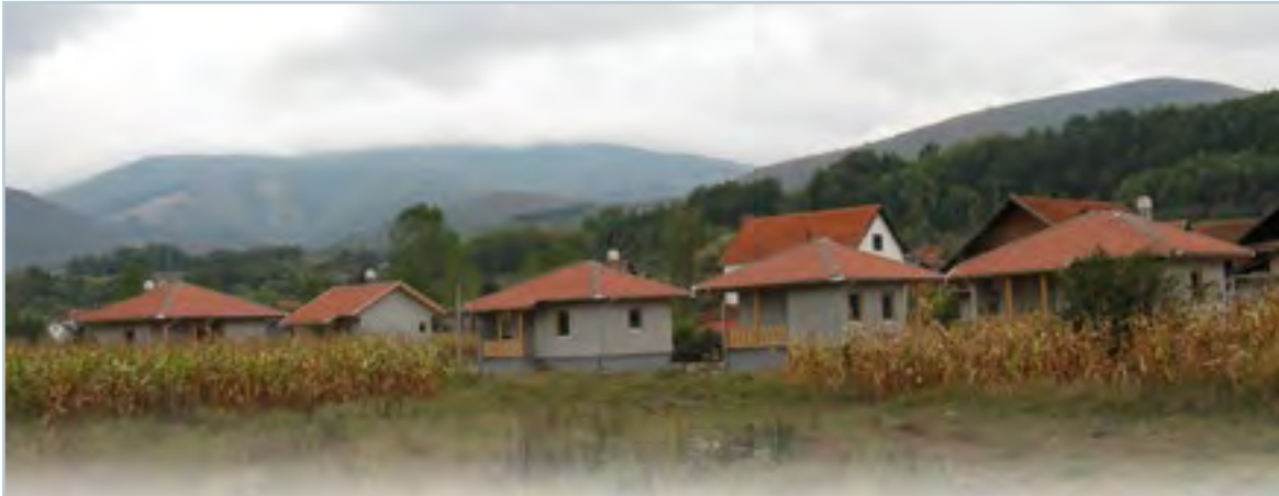
Prefabricated houses are built for refugees and internally displaced persons in Svrlijig. © IOM 2011
